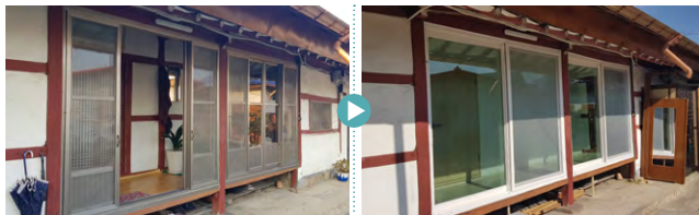
Photo of the house of Guk Jung-gwang before upgrading the windows
