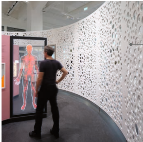
CNC milling machines routed various high-precision designs in the material
