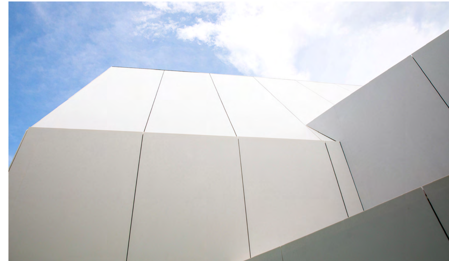
Design: Woo-jin, LIM AEV Architectures | Foto: AEV Architectures
